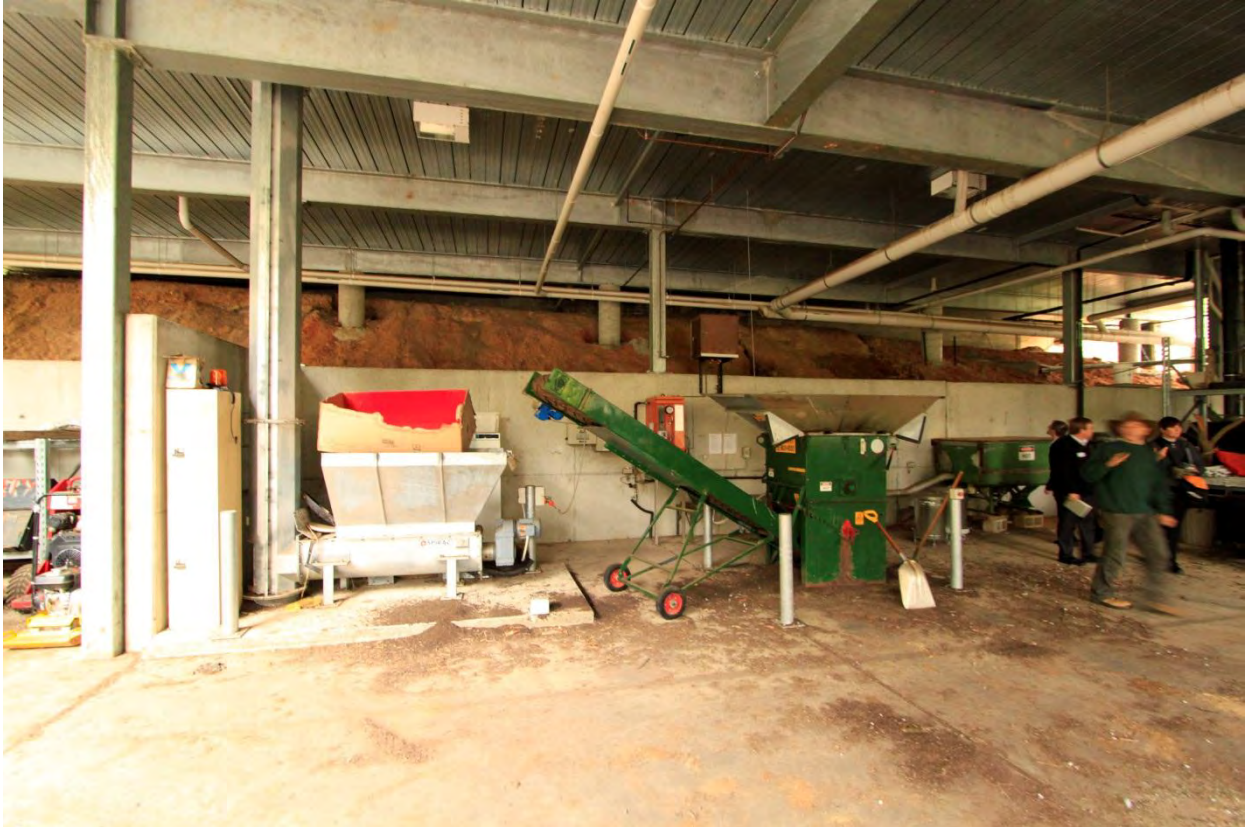
Figure 2 Existing Nursery Undercroft Area Media Mixing Machine
